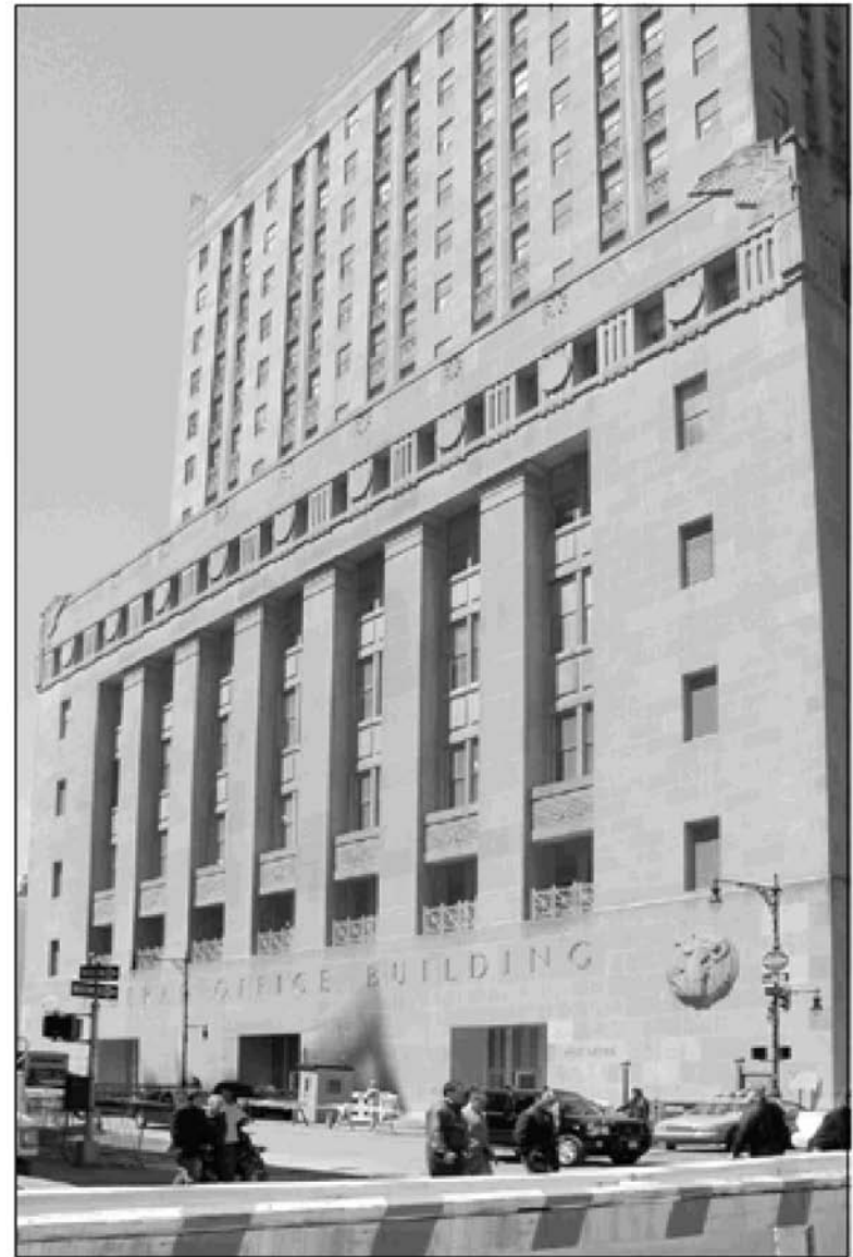
Federal Office Building/U.S. Post Office, 90 Church Street (2003)
