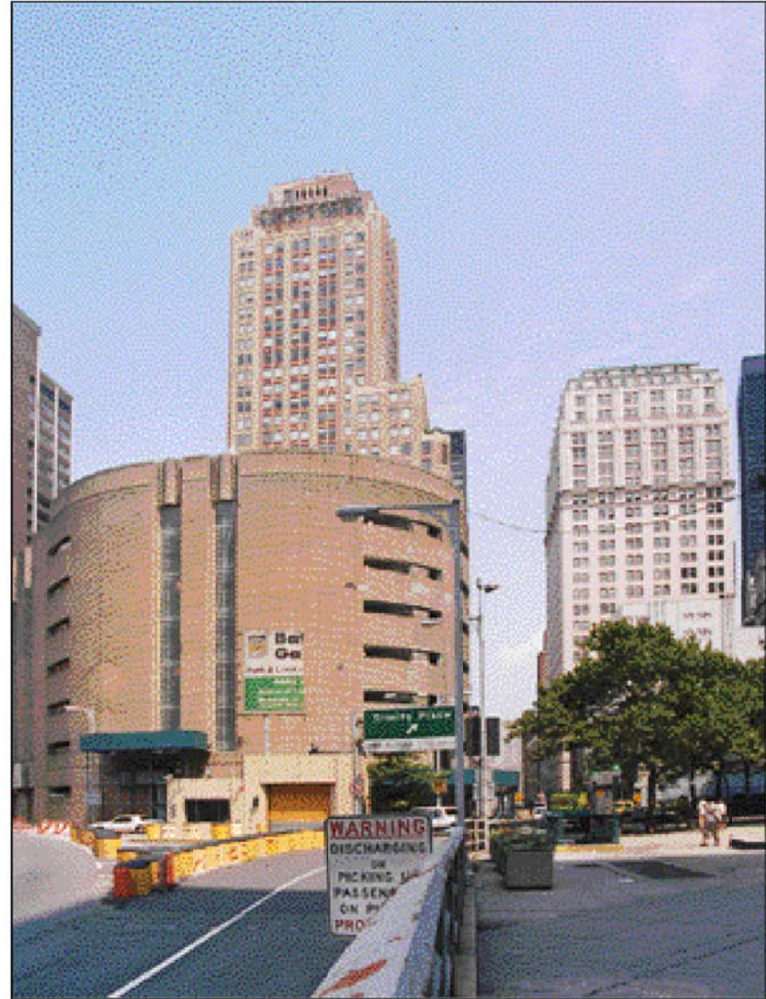
From left: Battery Garage at 56 Greenwich Street, 19 Rector Street (behind the garage) and the former Electric Bond and Share Company Building at 2-8 Rector street (right of garage) (2003)
