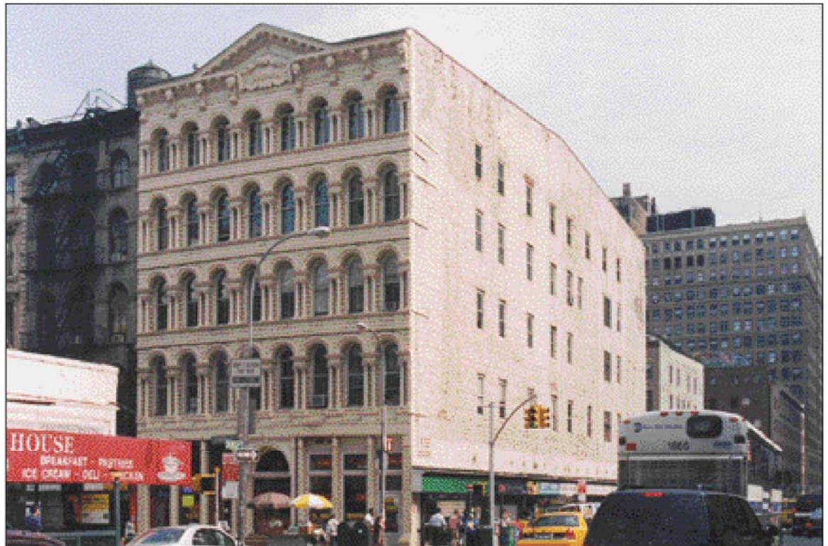
Cary Building, 105-107 Chambers Street (2003)
